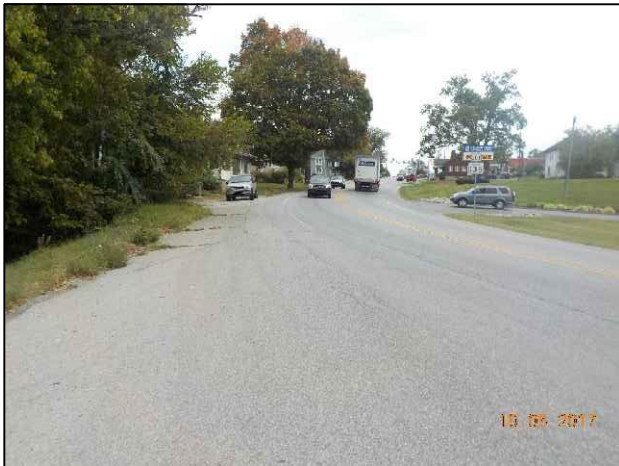
51. View of S.R. 56 near Mill St, looking northeast.
