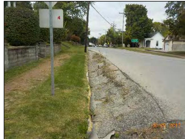
36. View of S.R. 56 near Posey St, looking west.
