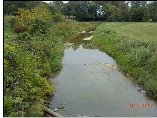
42. View of Brock Creek looking north (upstream) from S.R. 56.
