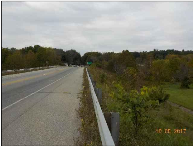
3. View of S.R. 56 looking southwest.
