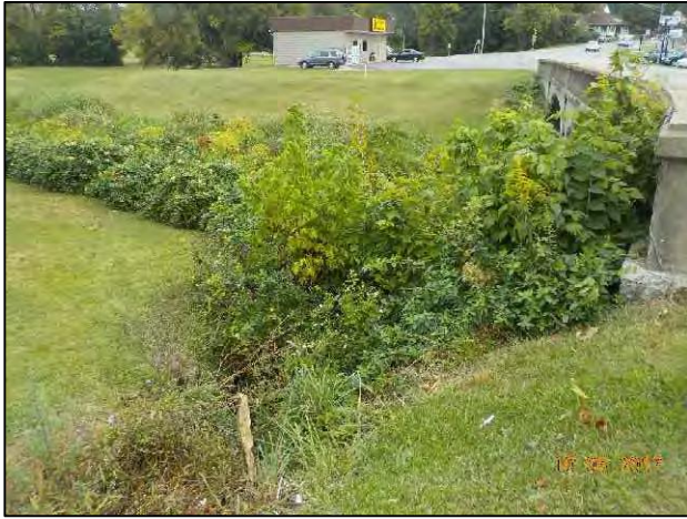
41. View of RSD 4, flowing into Brock Creek, looking northeast.
