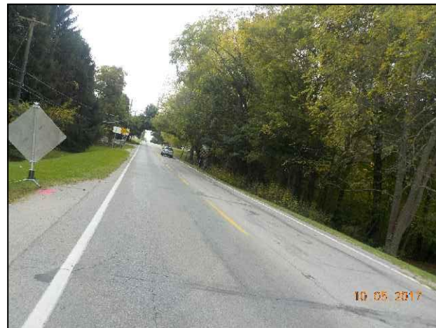
84. View of S.R. 135 near UNT 2, looking south.
