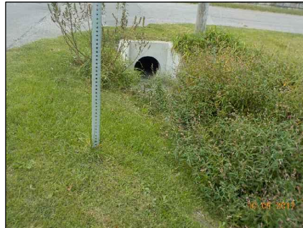
40. View of RSD 4 looking west.
