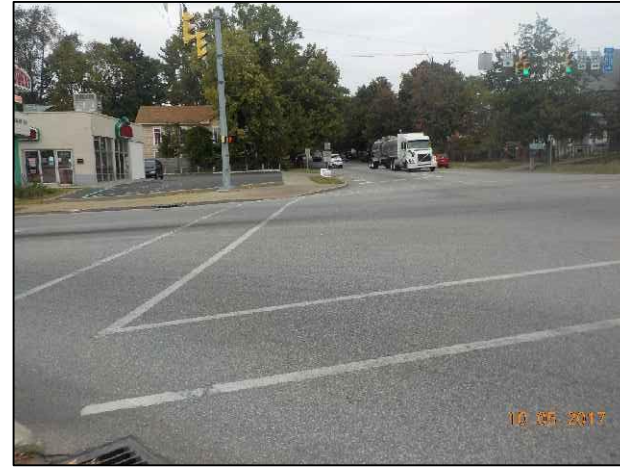
54. View of intersection of S.R. 56 and S.R. 135, looking north.
