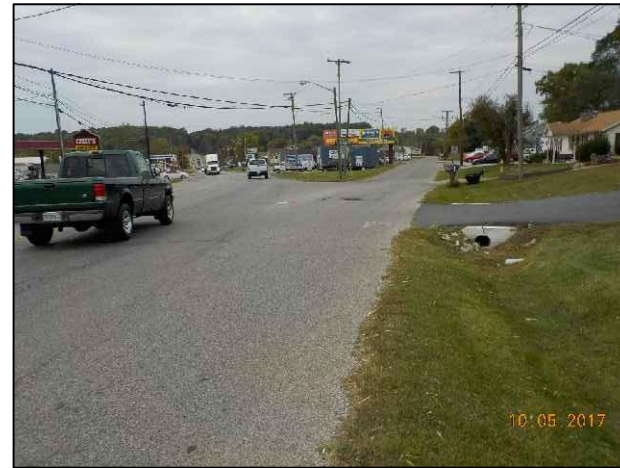
16. View of S.R. 56 and RSD 2 looking southwest.
