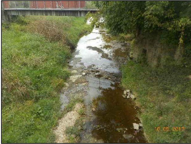
45. View of Brock Creek looking south (downstream) from S.R. 56.
