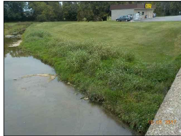
44. View of eastern bank of Brock Creek looking northeast from S.R. 56.
