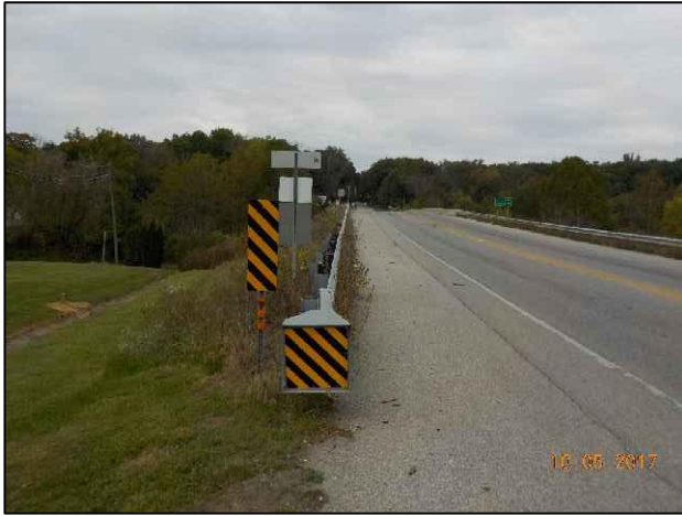
1. View of S.R. 56 looking southwest.
