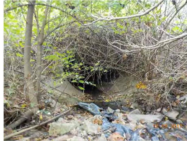
6. View of culvert carrying UNT 1 beneath S.R. 56, looking northwest.
