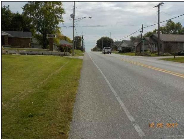
27. View of S.R. 56 looking southeast.
