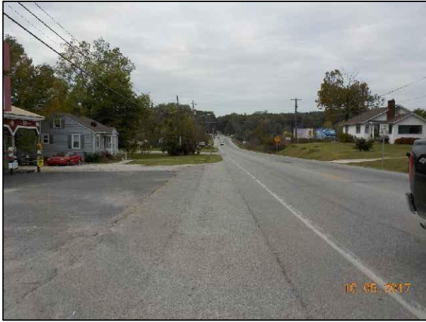
9. View of S.R. 56 looking southwest.
