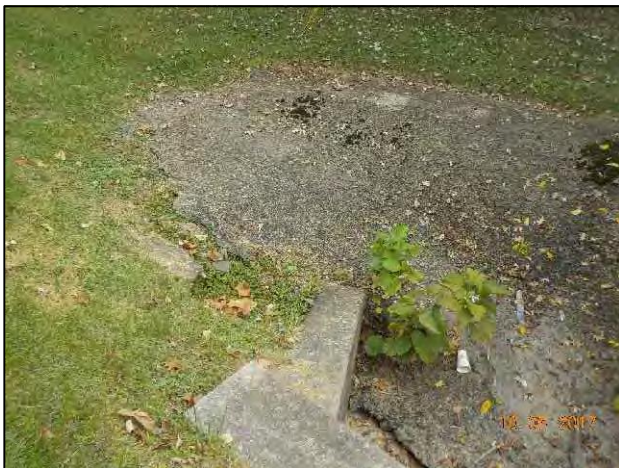
79. View of northern bank of UNT 2 from S.R. 135, looking northeast.
