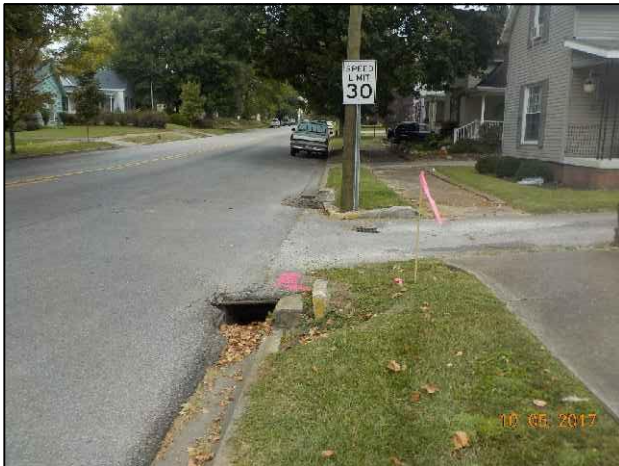
63. View of S.R. 135 looking north.
