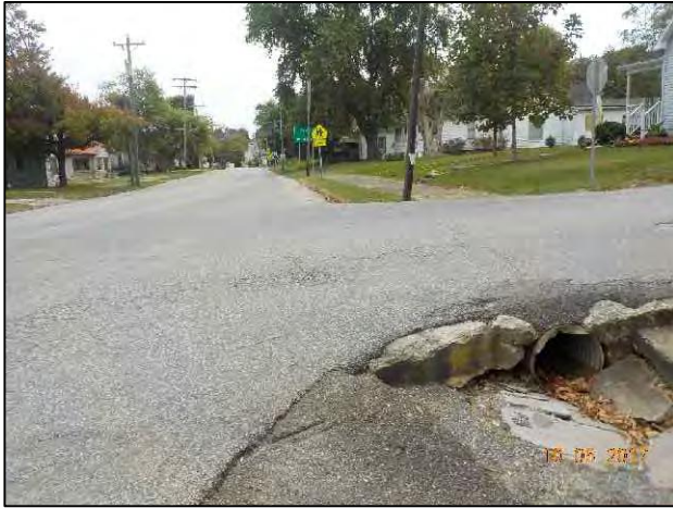
33. View of intersection of S.R. 56 and Shelby St, looking east.
