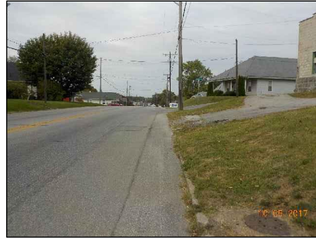
30. View of S.R. 56 looking northwest.
