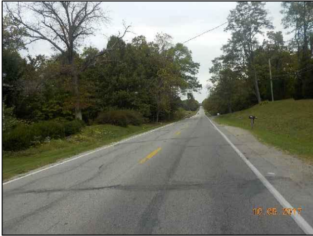
85. View of S.R. 135 near UNT 2, looking north.
