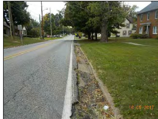
72. View of S.R. 135 near Reid Ave, looking south.
