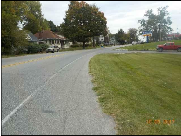
49. View of S.R. 56 near Mill St, looking northeast.
