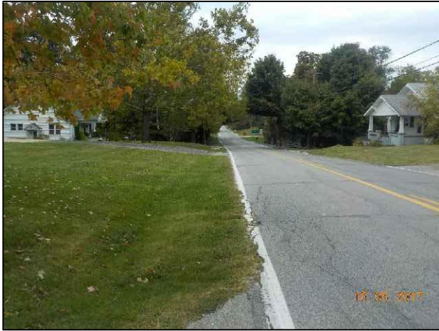
77. View of S.R. 135 near Emma St, looking north.
