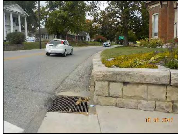
38. View of S.R. 56 near Posey St, looking west.
