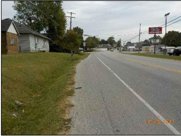
21. View of S.R. 56 and RSD 2, looking east.
