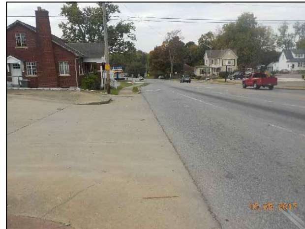
52. View of S.R. 56 near S.R. 135, looking west.
