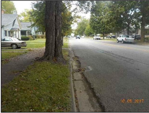
65. View of S.R. 135 looking north.
