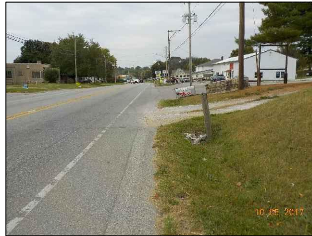
20. View of S.R. 56 and RSD 2, looking west.
