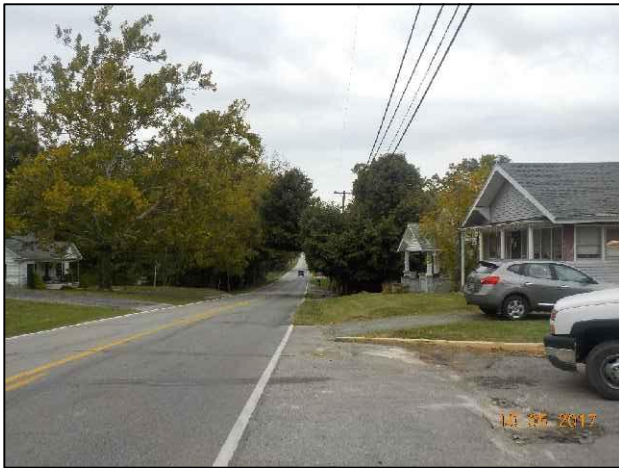
75. View of S.R. 135 near Emma St, looking north.
