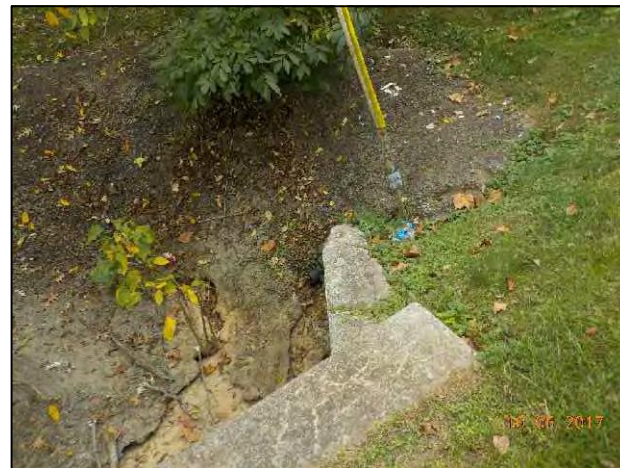
80. View of southern bank of UNT 2 from S.R. 135, looking southeast.
