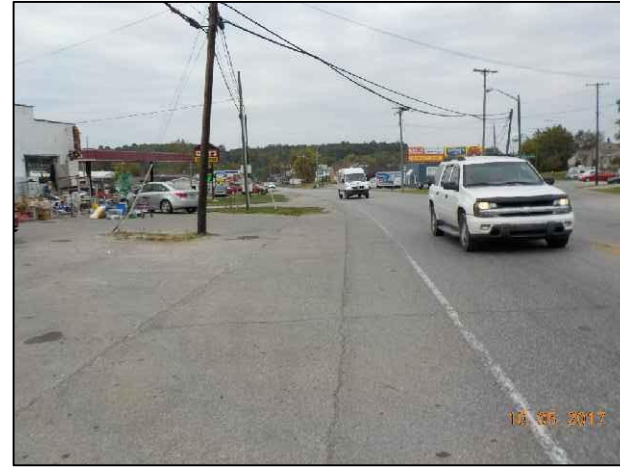
14. View of S.R. 56 looking southwest.
