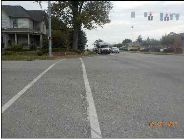
57. View of intersection of S.R. 56 and S.R. 135, looking east.
