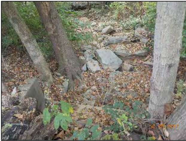
81. View of UNT 2 from S.R. 135, looking west.
