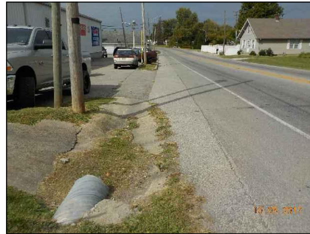
24. View of S.R. 56 and culvert, near Marshall Ave, looking northwest.
