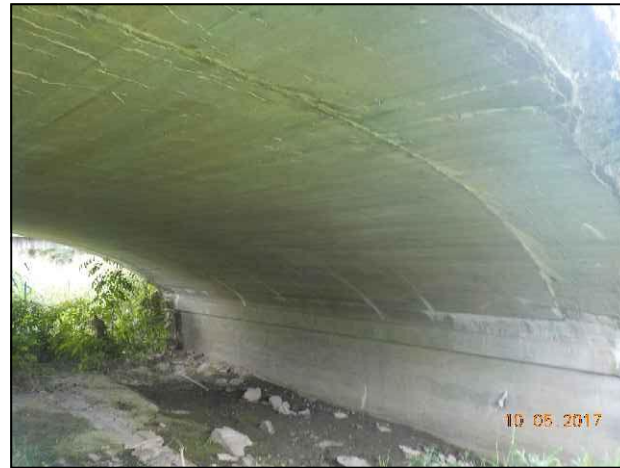
92. View beneath S.R. 56 bridge looking south.
