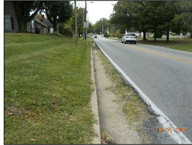
70. View of S.R. 135 near Reid Ave, looking south.
