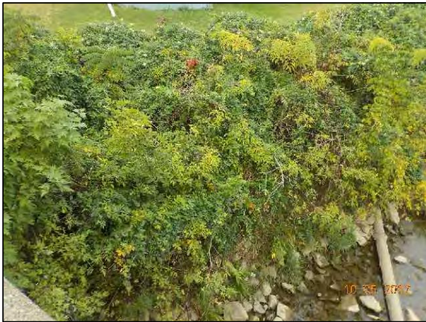
43. View of western bank of Brock Creek looking northwest from S.R. 56.
