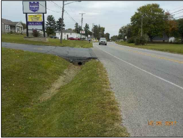
17. View of S.R. 56 and RSD 2 looking northeast.
