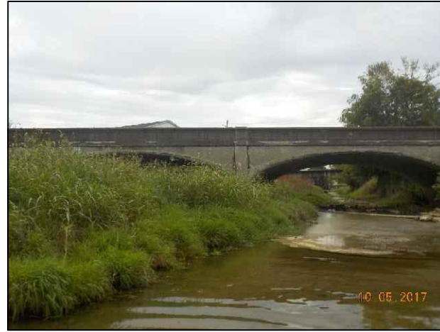
90. View of Brock Creek and S.R. 56 bridge looking south (downstream).
