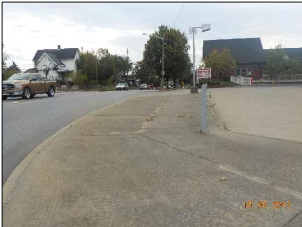
55. View of S.R. 135 looking south from S.R. 56 intersection.
