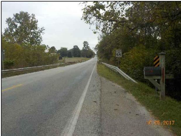
87. View of S.R. 135 from northern project boundary, looking north.
