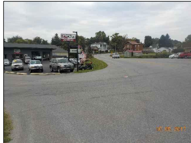
48. View of intersection of S.R. 56 and Mill St, looking southwest.
