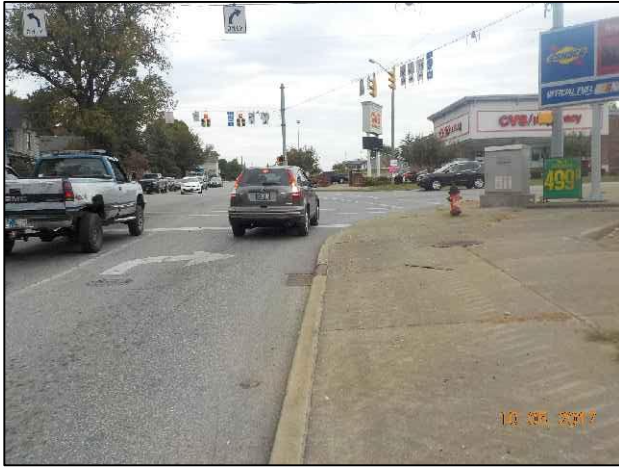
53. View of S.R. 56 near S.R. 135, looking east.
