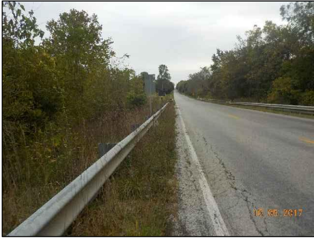
89. View of S.R. 135 from northern project boundary, looking north.
