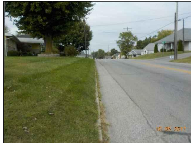
28. View of S.R. 56 looking northwest.
