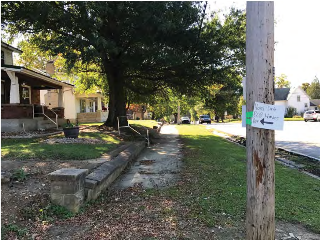
6. Looking south at sidewalks starting at Homer Street
