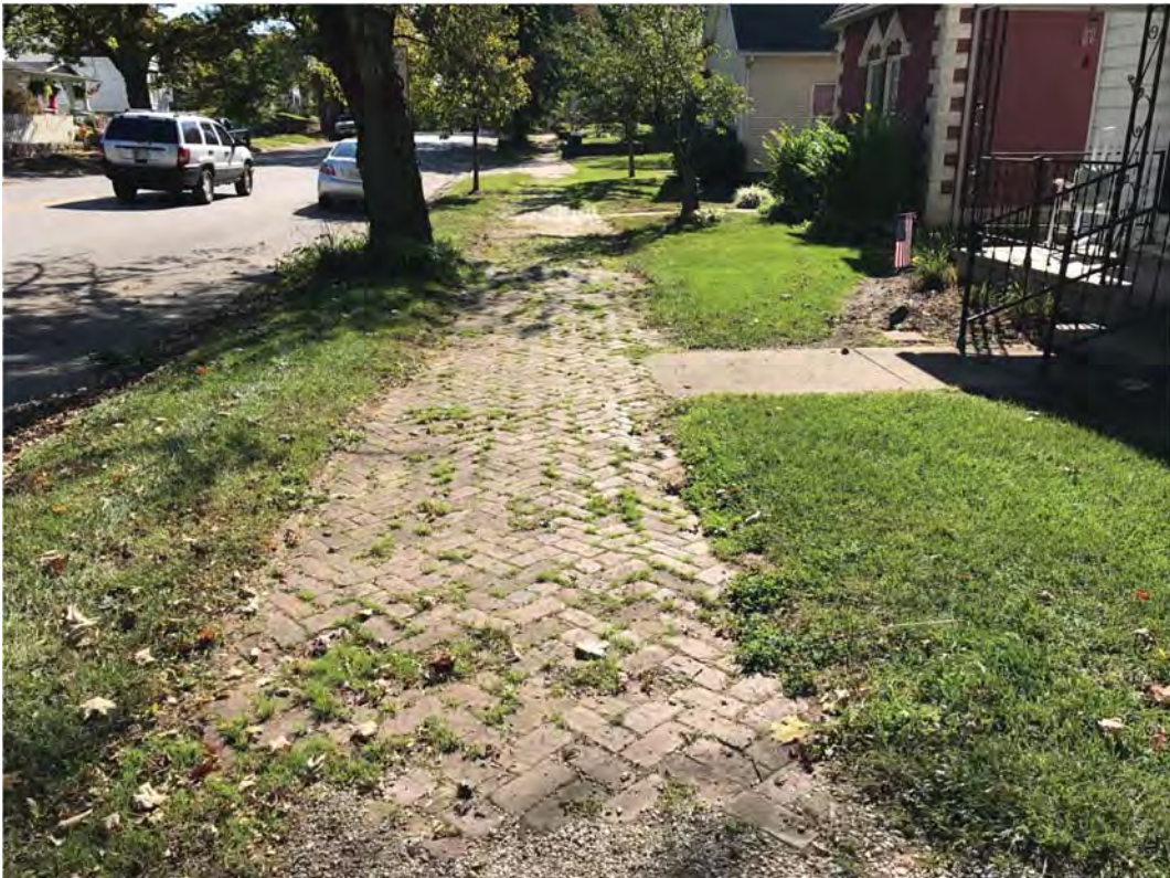
10. Looking south at herringbone pattern brick sidewalk, west side of 600 block North Main
