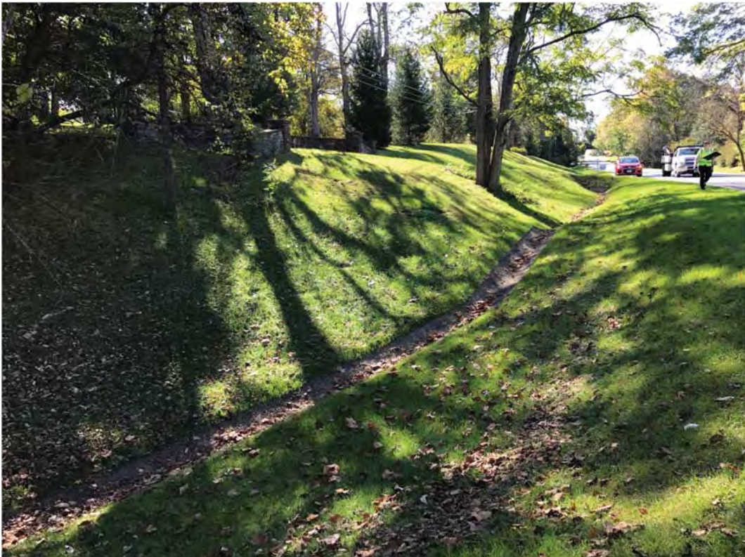
2. Looking south at concrete ditch on property of 1201 Main St., G-2
