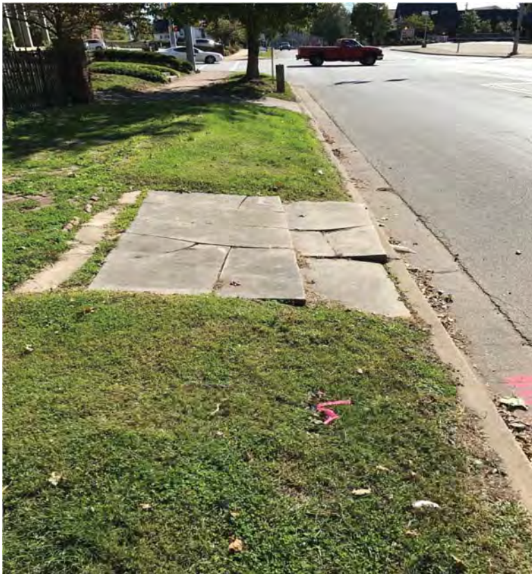
19. Looking south at stone slab steps in front of N. 401 Main
