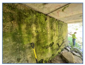
Photo 8: Looking southwest under Structure #06-00061 at staining on south abutment (6/1/23).
